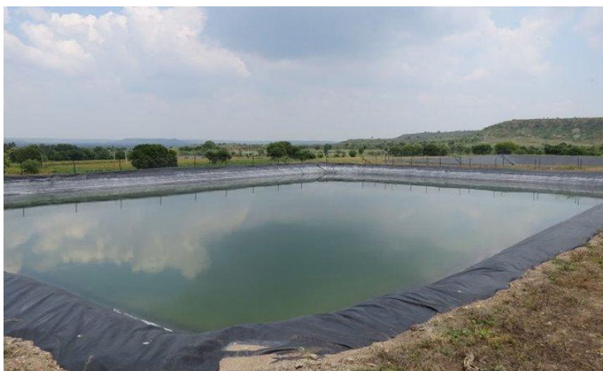
Figure 3. 6: Farm ponds / Percolation ponds
