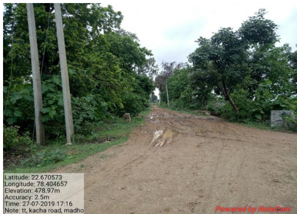
Figure 5- 33: Existing Situation of Roads
